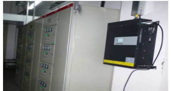
Wall mounting in power distribution room
